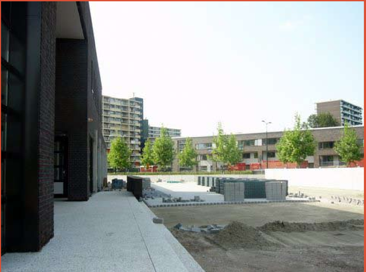
The front of the church. The surrounding housing estate is the new field for harvest.
