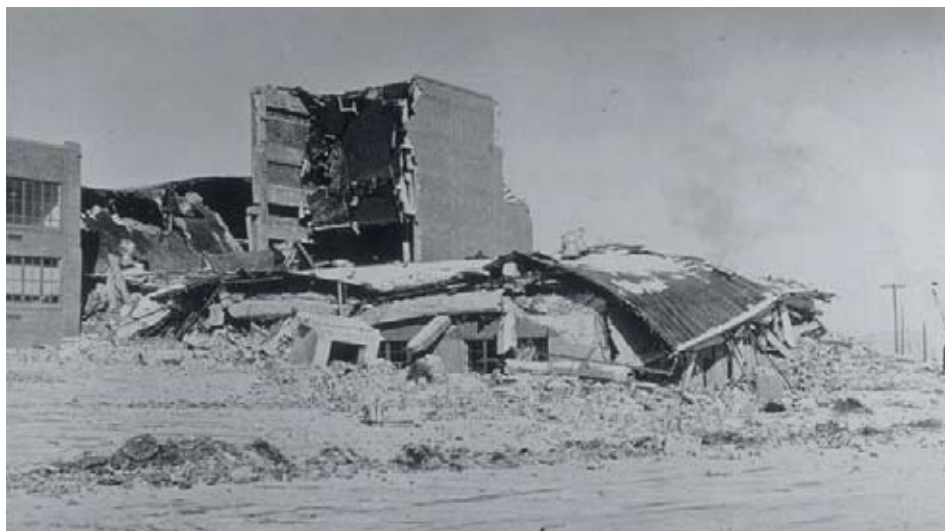
The west wing of the new Helena High School lay in ruins after a second major quake in two weeks on Oct. 31, 1935. http://montanayesterday.com
