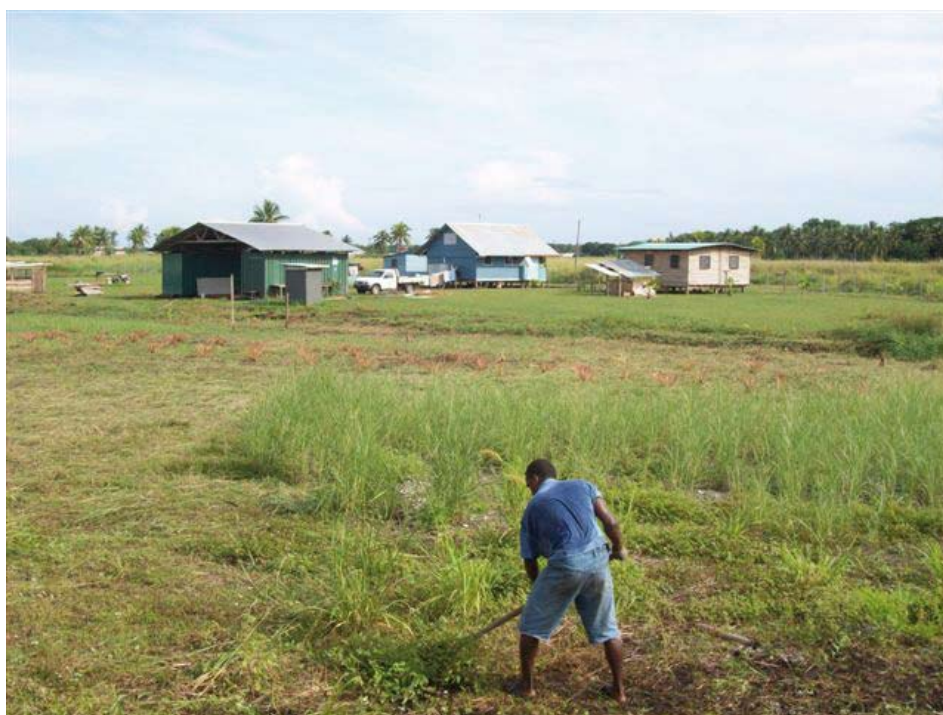
Building progress at Bethesda Centre
