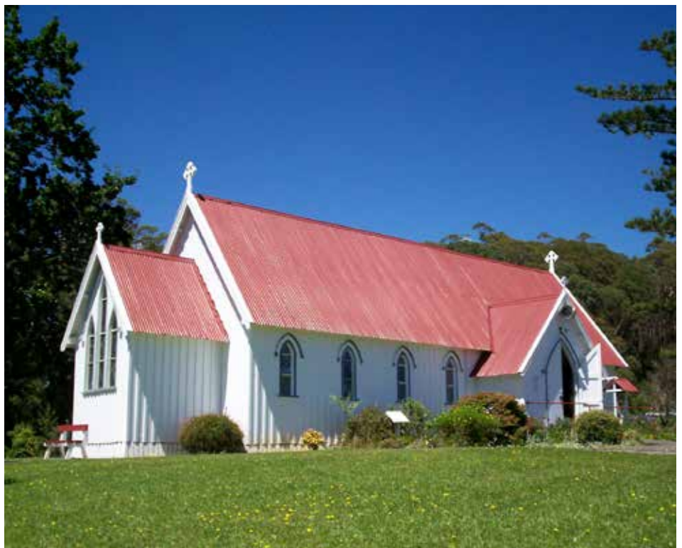
St James Church in Kerikeri, one of the many churches built with the expansion of the gospel.
